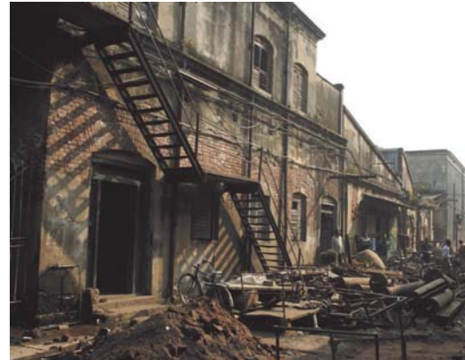
Interior of the India Jute Mill.
