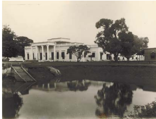
1934. The water tank with the government house behind (MMD).
