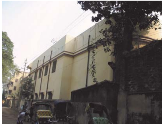
2009. Condition of the church.
