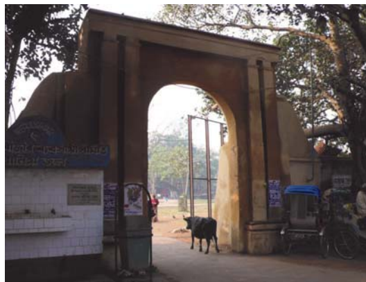
2009. The main gate behind a public drinking water service and local rickshaws.
