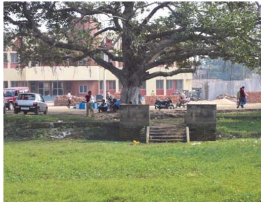
2009. The overgrown water tank.
