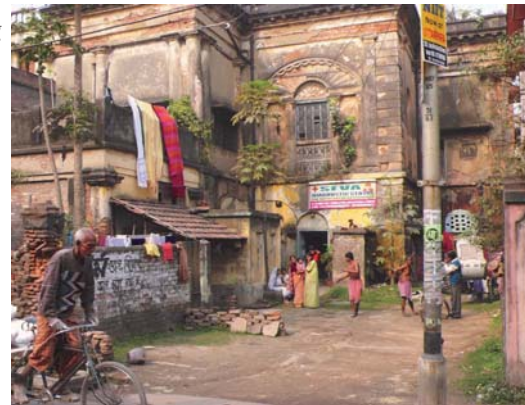
2009. Condition of the building on T. C. Goswami St. 30.
