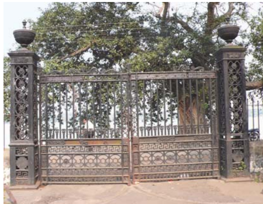
Condition of the main gate.
