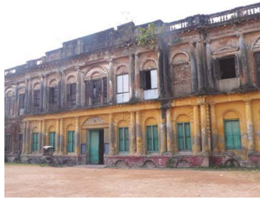
2009. The main façade of the southern complex of the Rajbari.
