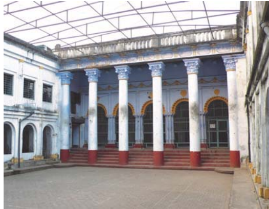
2009. Condition of some of the Dey residences on Dey Street.
