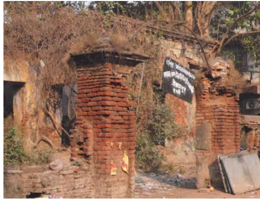
2009. Condition of the building on T. C. Goswami St. 29.
