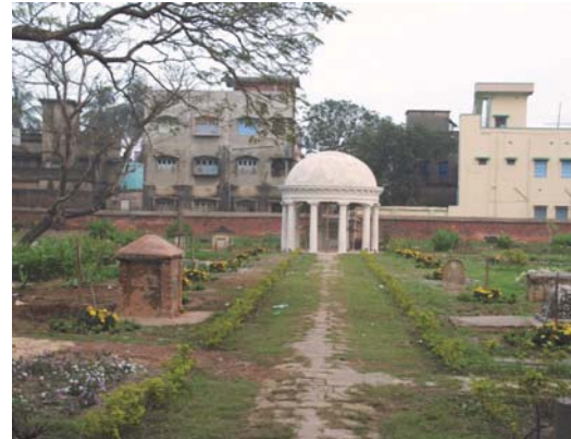
2009. The restored monuments of J. Marshman and W. Ward.
