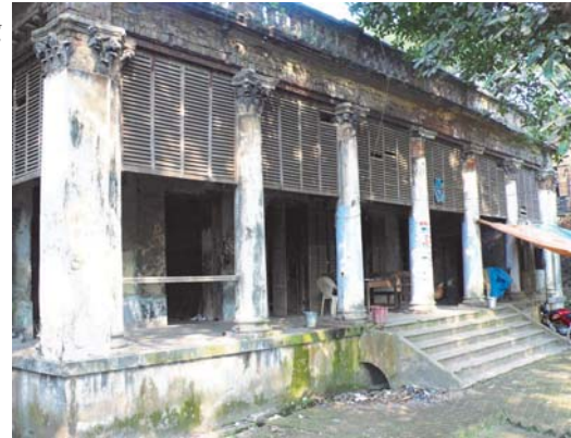
2009. Condition of the building on T. C. Goswami St. 31.
