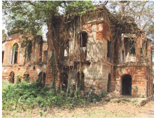
2009. Condition of the so-called Bore House on T. C. Goswami St. No. 22.
