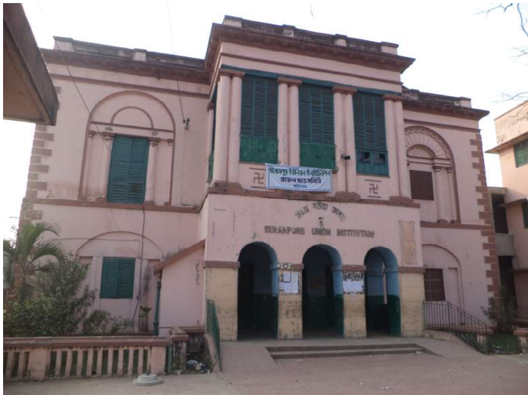
Serampore Union High School old building
