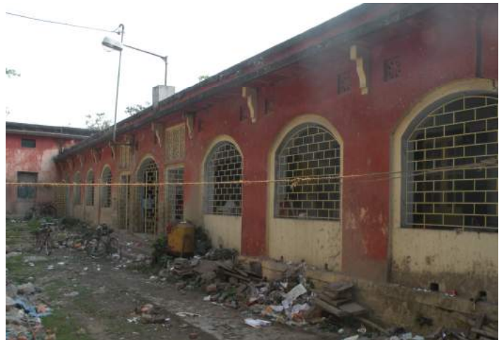
View of the east (rear) façade
