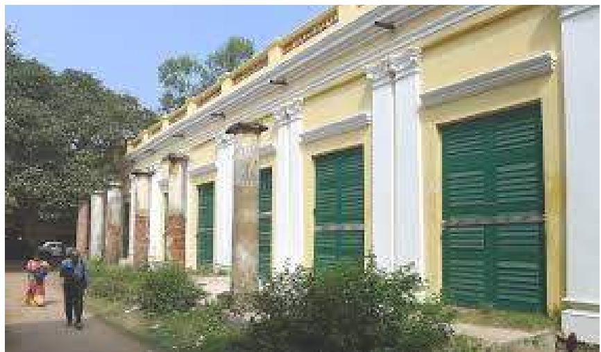
The South facade after restoration
