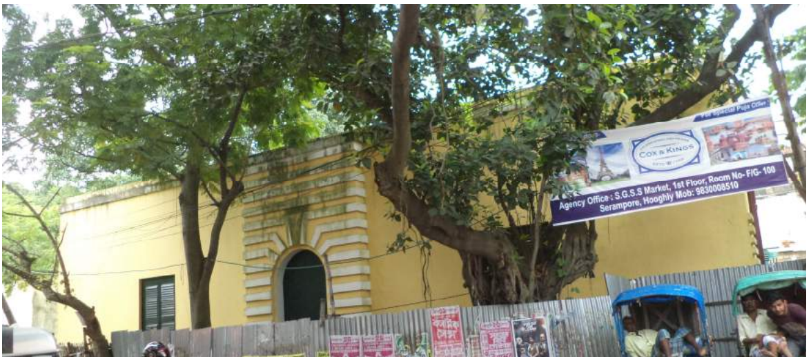
South façade after restoration in 2015
