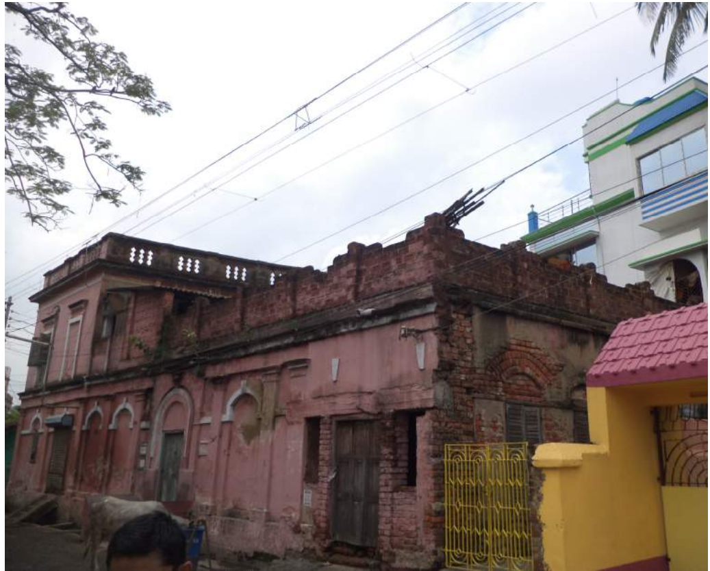
View from entrance
