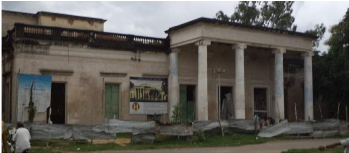
Danish Government House under restoration (2013)
